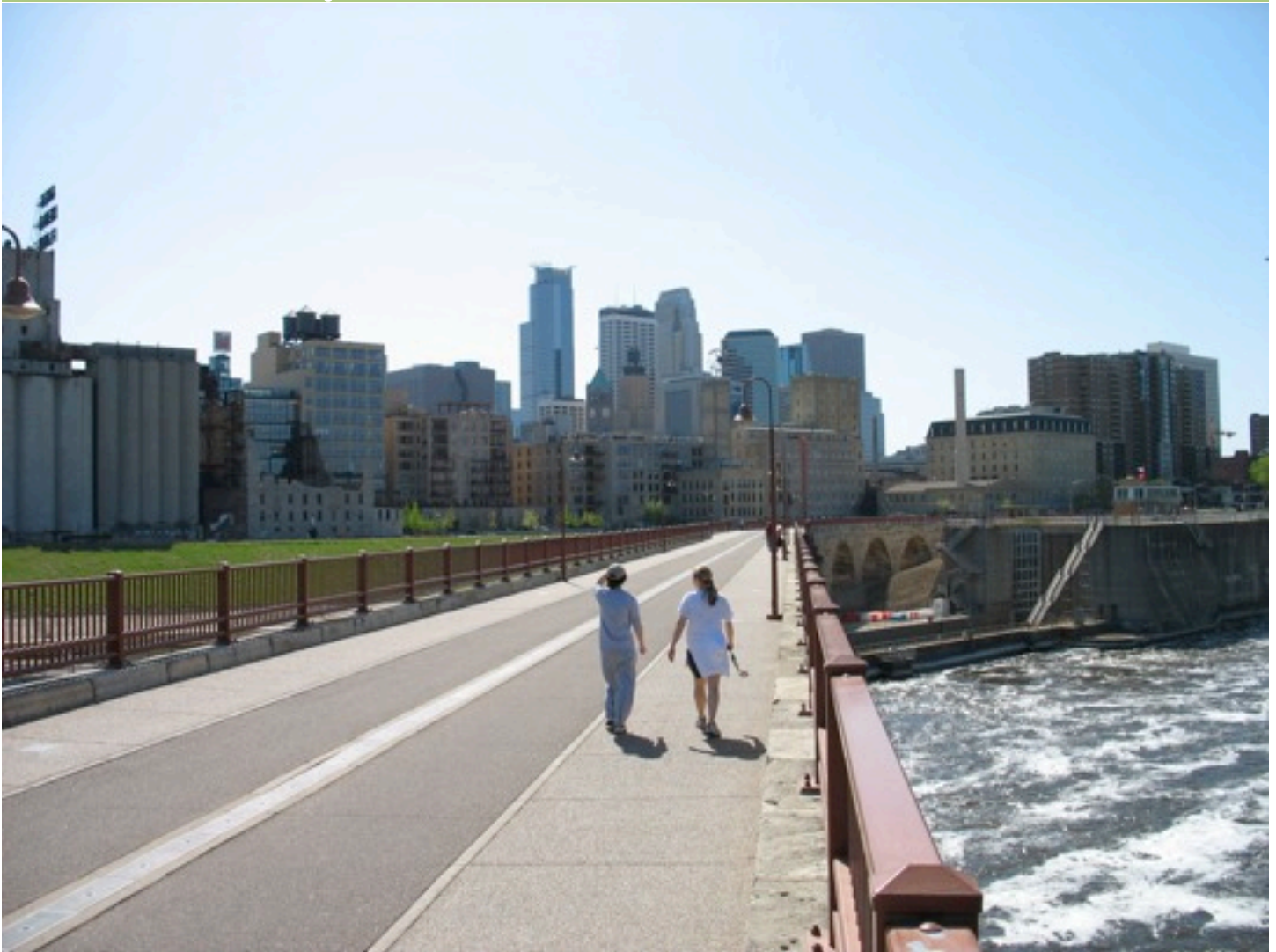
Minneapolis Stone Arch Bridge
